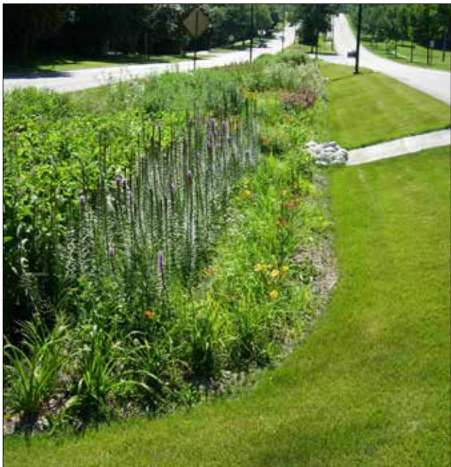
Naturalized swale enhancing infiltration
