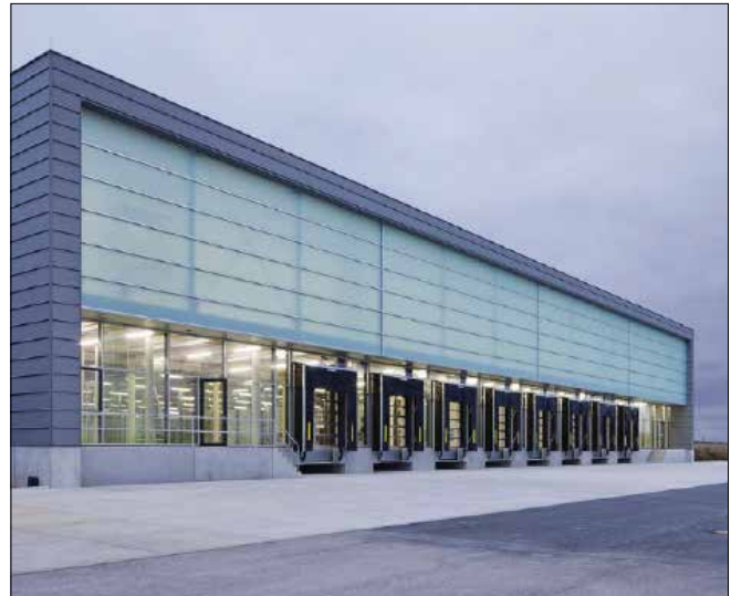
Loading bay defined by a recessed wall plane and glazing
