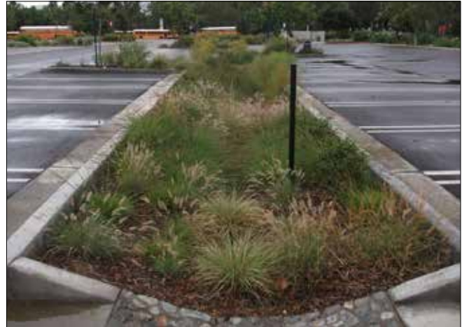
Planted island allowing surface water infiltration
