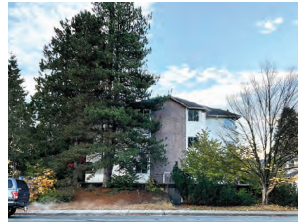
West Elevation Facing Harris Road
