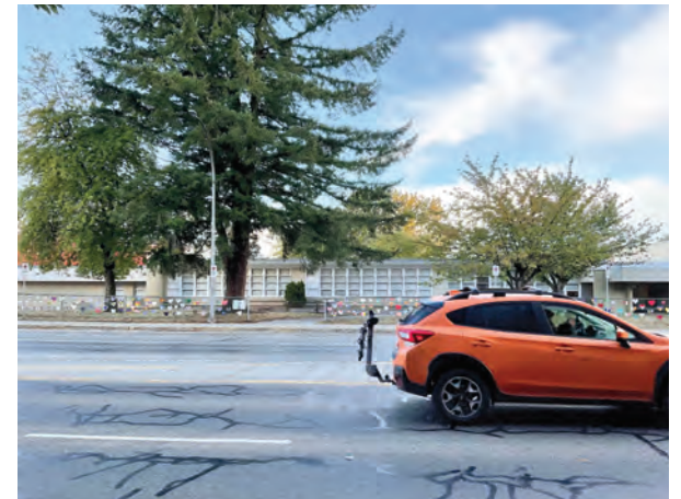
East Windows of Original 1953 Facade
