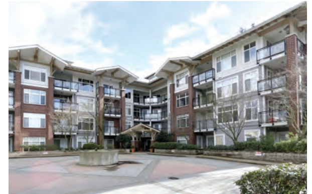
View from Courtyard
