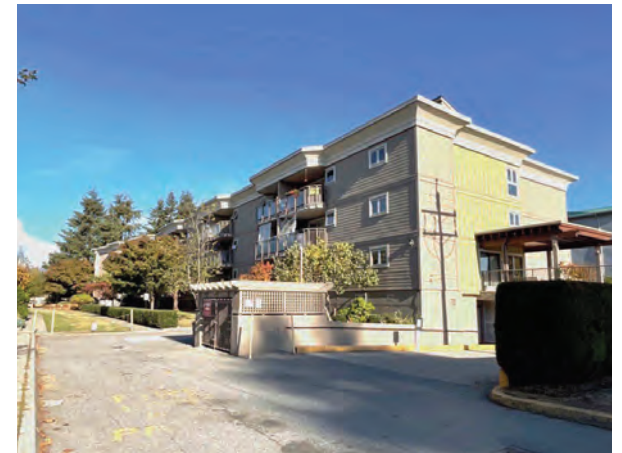
Truncated Parking Garage Entry at South Property Line
