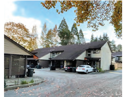
Unit along the Lane within the Complex
