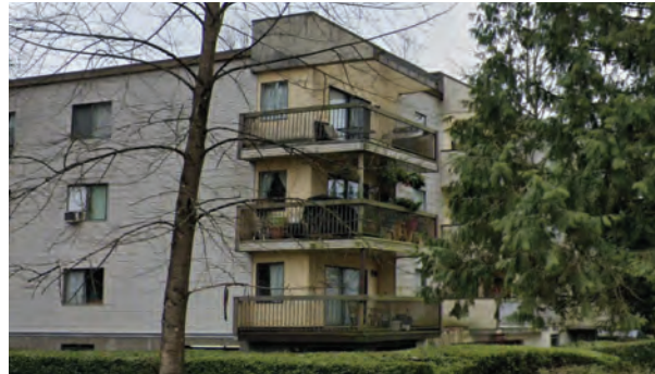
Street View from North East
