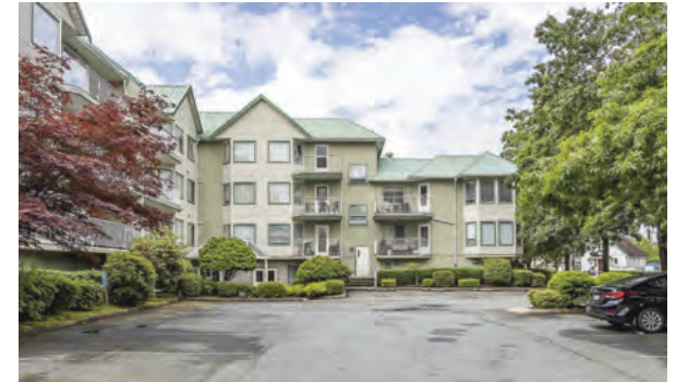
View of Partial East Elevation
