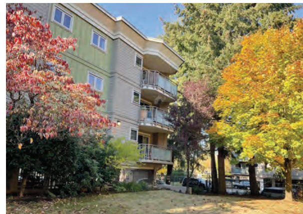
East Firelane. Parking Garage noted as being partially below grade
