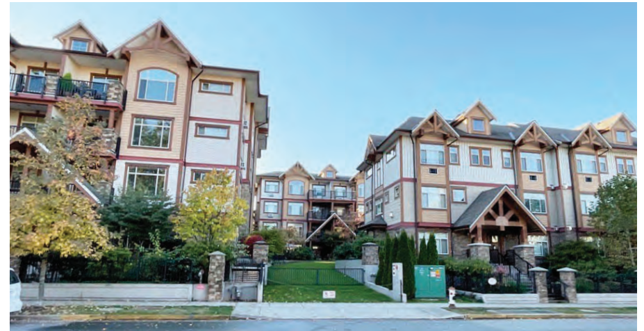
View of Fire Lane from East
