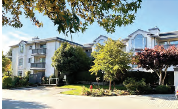
East Elevation of Overall Building Facade
