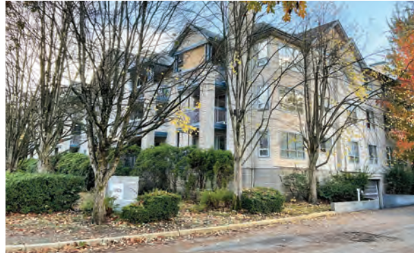
South West View from Harris Road
