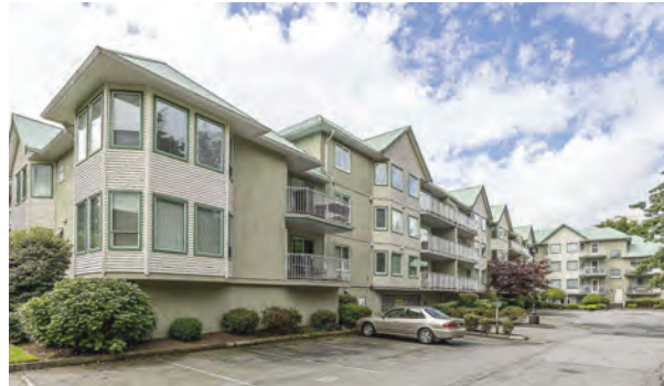
View from North East Corner
