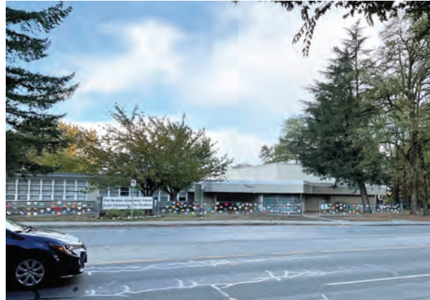
Main Entry along Harris Road
