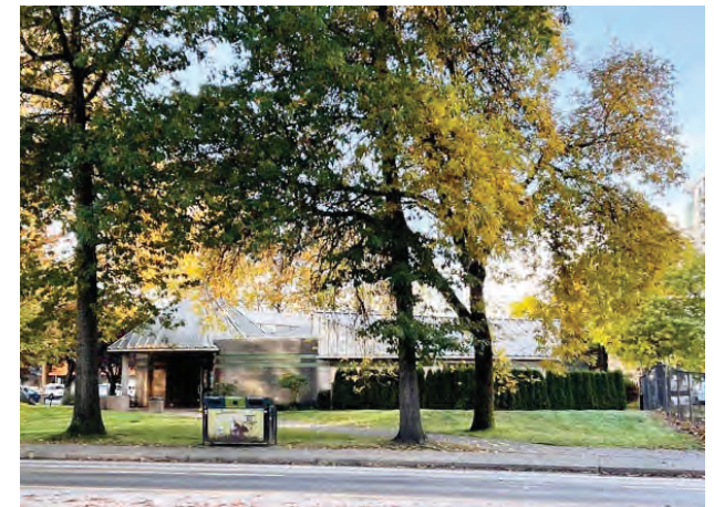
East View Street View of Auditorium from Harris Road
