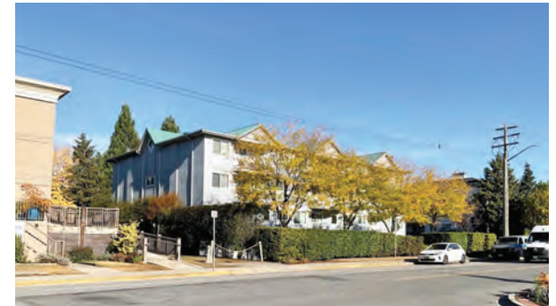
South West View
