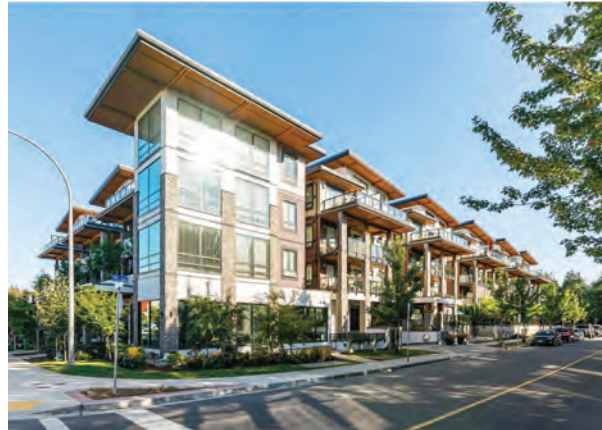
View from North West Corner
