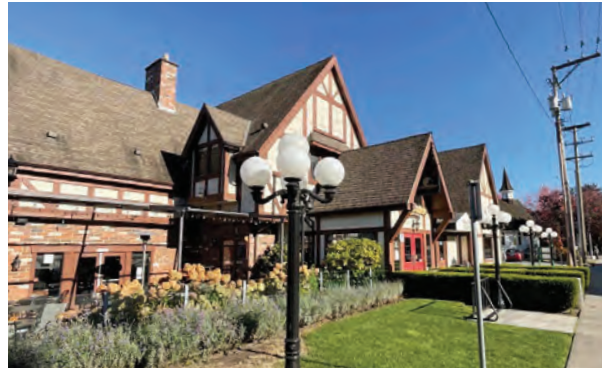
Southeast View of Main Entry
