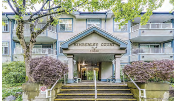
View of Entry from Harris Road
