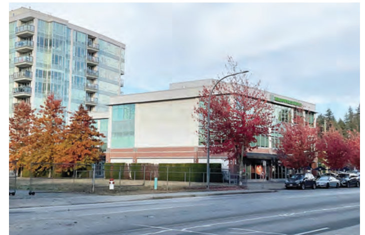
South East View from Harris Road
