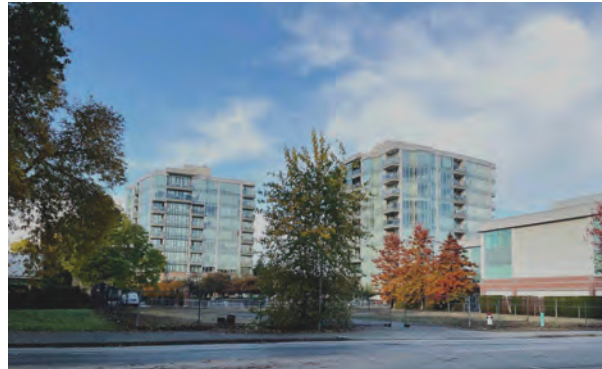
South East View from Harris Road
