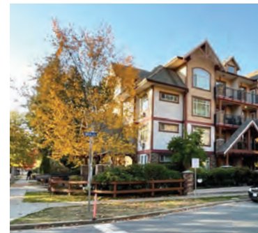
View from South East Corner
