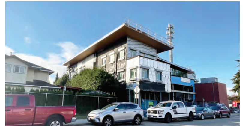
View of New Fire Hall under Construction
