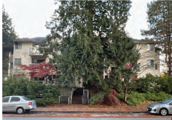
North Elevation and Entry
