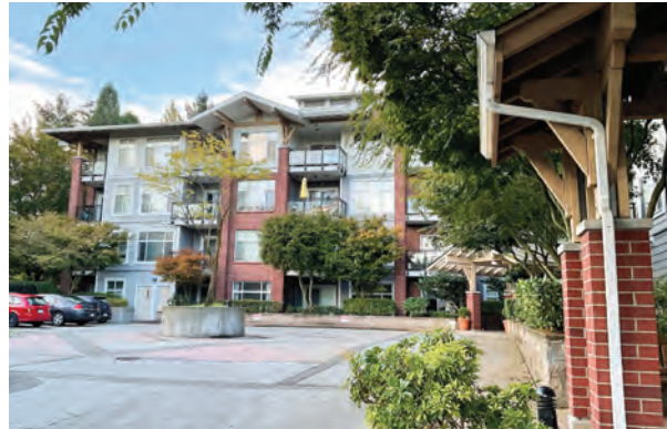
View of West Facade from Courtyard
