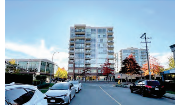
View of North Elevation
