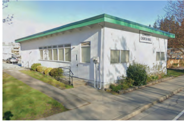
Northwest View of Church at Intersection of Harris Road and Ford Road
