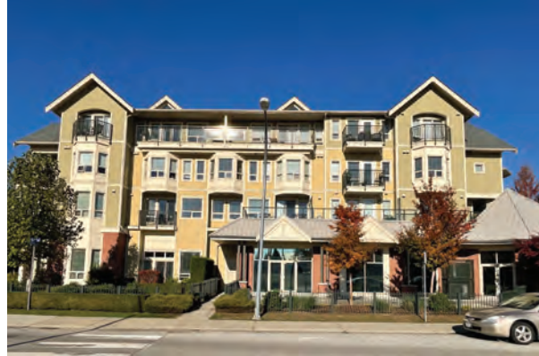
View of South Elevation
